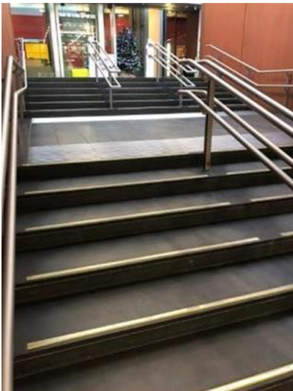
Image of steps from Hello Desk to lifts, with metal handles and white marking at the edge of each step.
