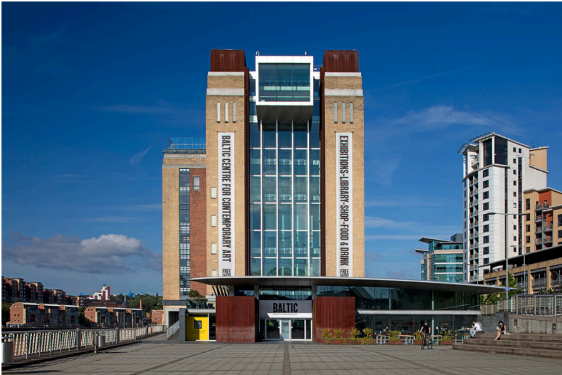
Photo: Baltic Building by Graeme Peacock
