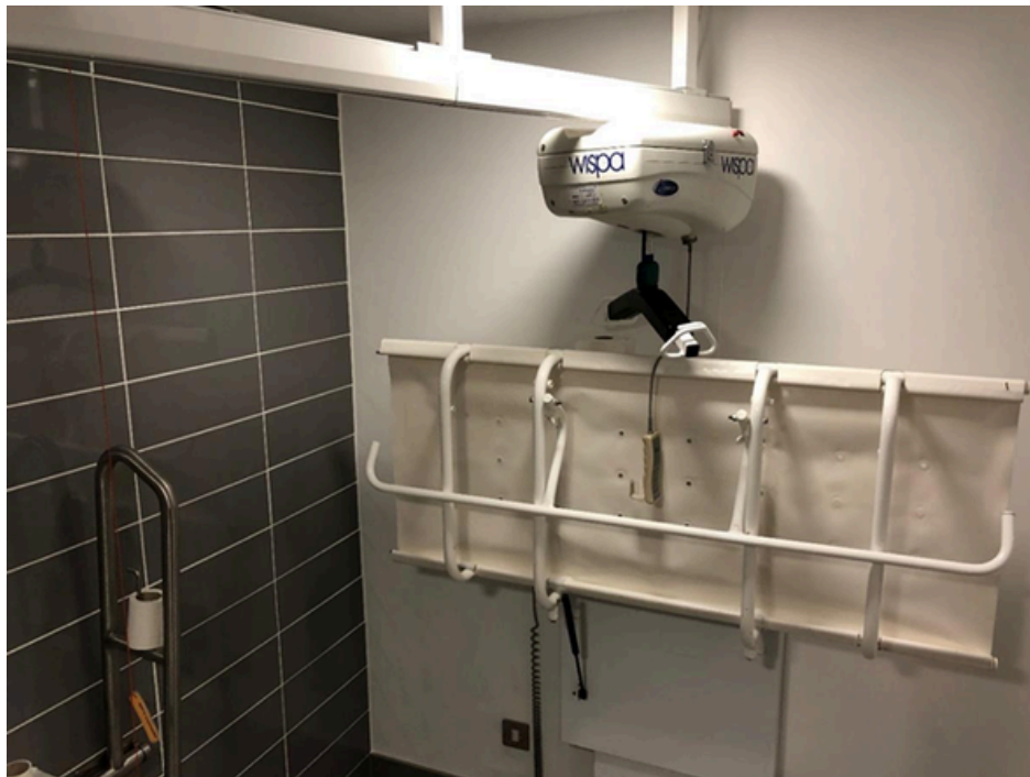
Image of ground floor access changing room with hoist and fold down bed, toilet with height adjustable sink
